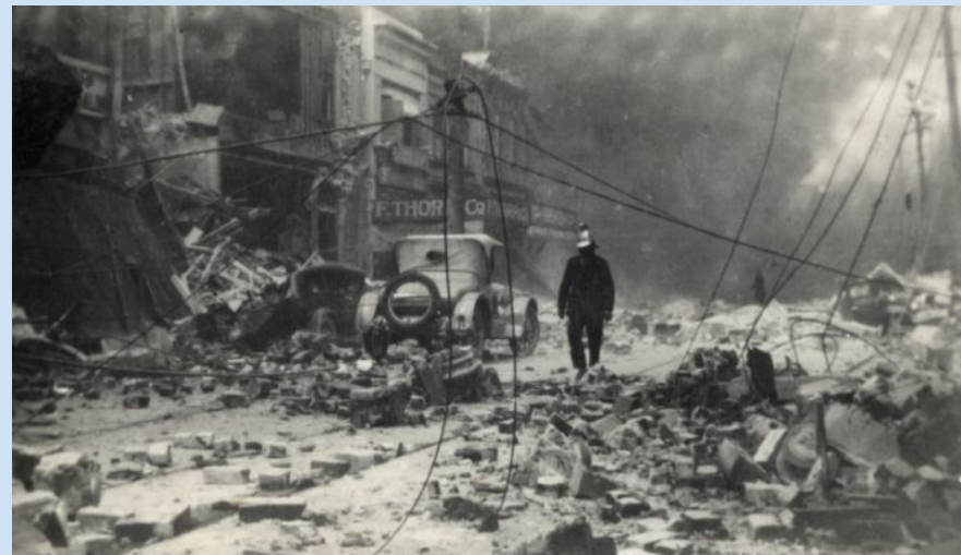
This is a street that had lots of damage done to it after the earthquake.
