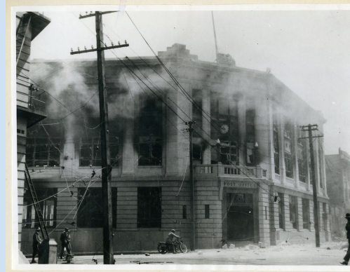
This building caught on fire after the earthquake had happened.
