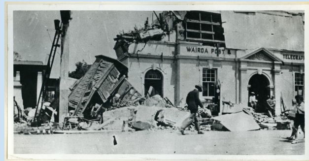
One of the damaged buildings in Napier after the earthquake.
